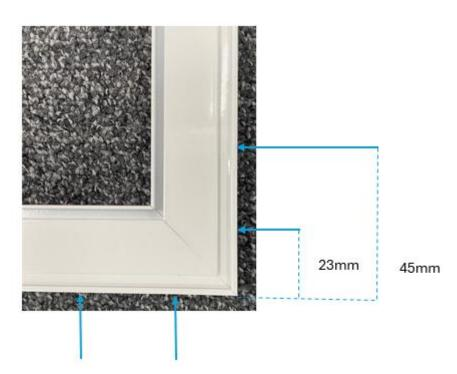
one 23mm from the corner and another 45mm from the corner. Make sure the drill bit goes in to a depth of 1". Insert and screw in the No. 4 34" screws provided. See image below.
